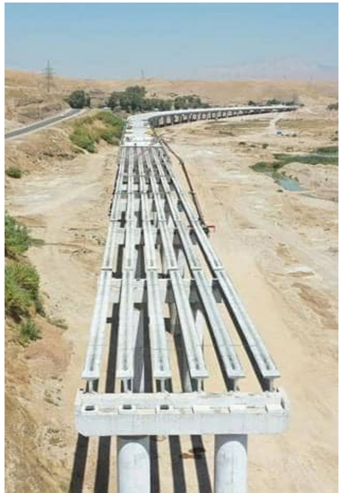
Highway construction between Sulaimaniyah and Germian
