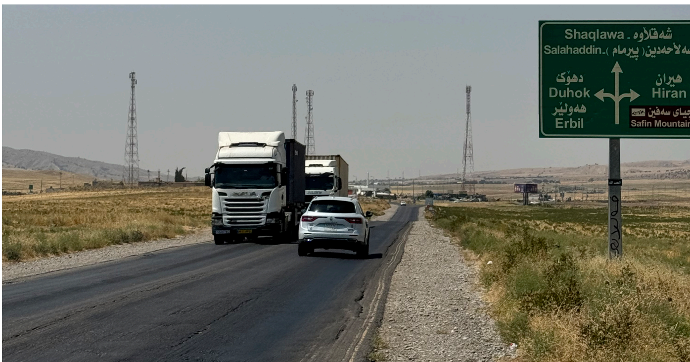
The highway between Erbil and Koya.
